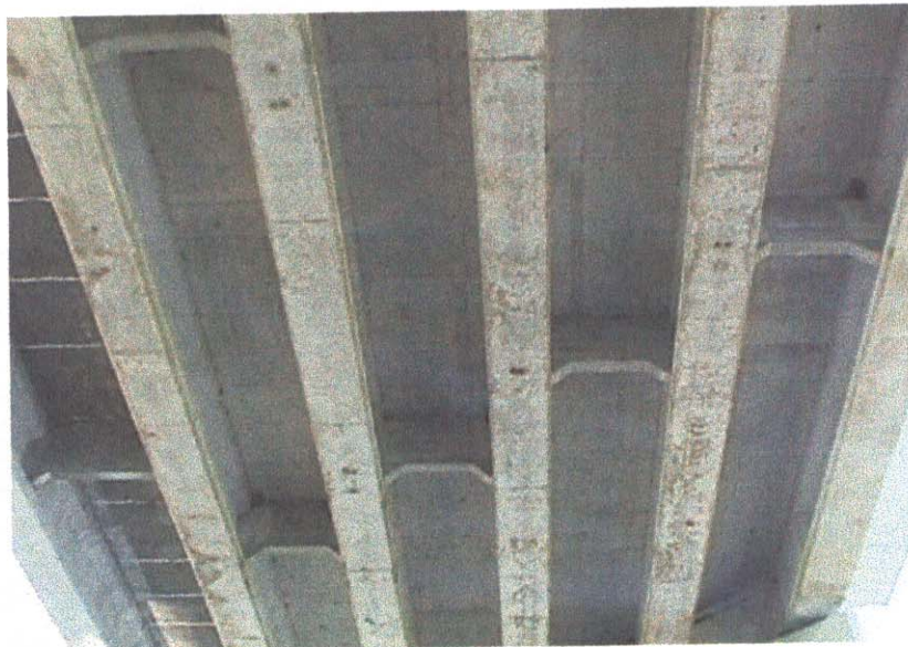
BOTTOM OF DECK
